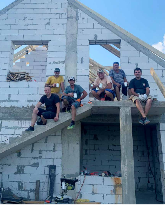
Above: Taking a well-earned tea break while working on Casa David. Above, right: 'S' demonstrating one of many building techniques.
